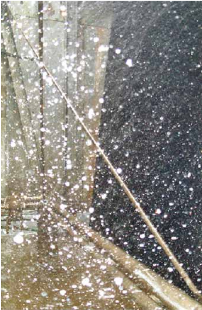
Figure 2: Cooling Tower Drift
