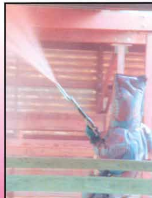
Spray Technician applying red dye colored preservative.
