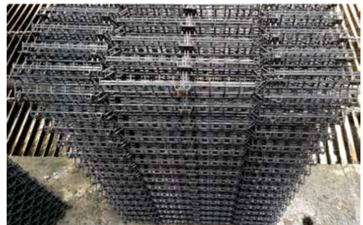
Figure 15: A Vertical Offset Modular Splash Fill pack still in service in a field installation.
